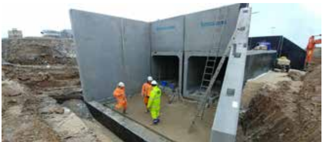
Box culvert with wing walls
